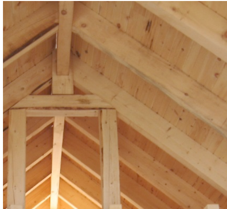
Figure 4 - Roof panel, inside view (ceiling)
