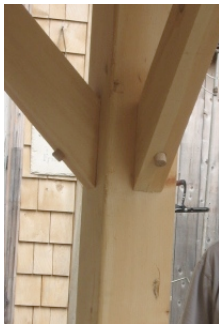
Figure 1- Hidden metal connector
