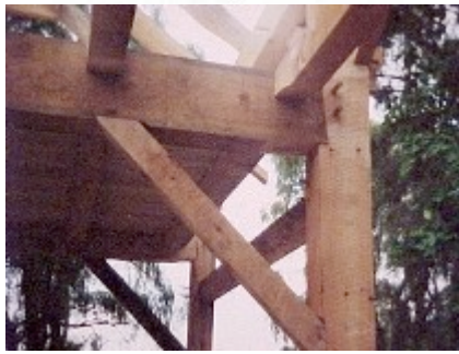
Figure 2-Traditional tenon & Mortise connection
